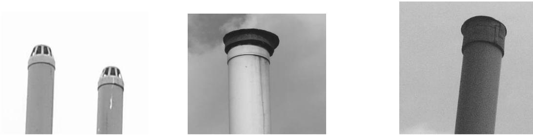
Figure 6.4.: Various rain shelters applied on vent pipes. Left picture represents a cover fitting in Bubaale, Kisoro Rd.; Middle image shows a combination of a cover fitting and a self constructed top piece; Right picture indicates a self construction without any space between the pipe and the shelter.
