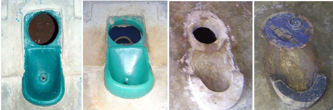
Figure 6.5.: Squatting pans. (f.l.t.r.) 1<sup>st</sup> and 2<sup>nd</sup> picture: Plastic pans in Kalungu. 3<sup>rd</sup> picture: Concrete pan in kisoro. 4<sup>th</sup> picture: Concrete pan with a lid in Kisoro.
