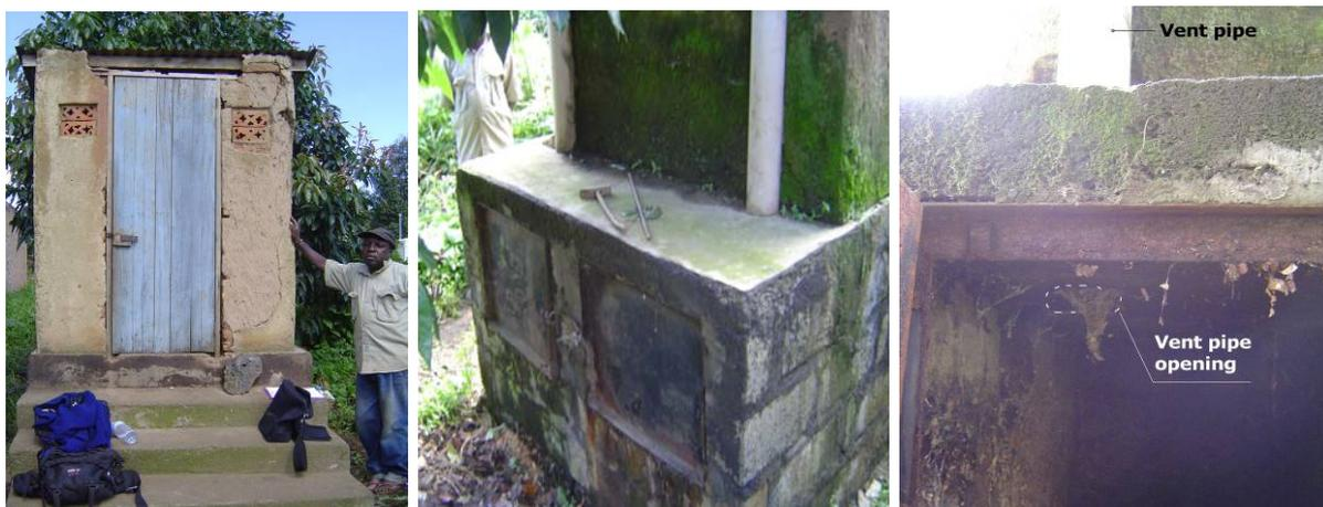
Figure 6.10.: (f.l.t.r.) Front view. Rear view (vertical doors; two outside vent pipes. Detail of the left chamber (vent pipe breakthrough)
