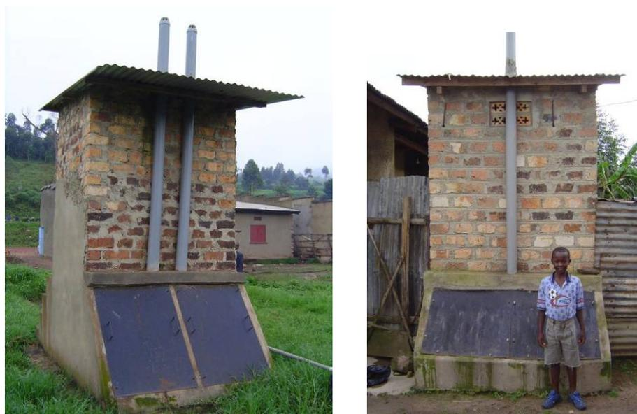
Figure 6.3.: Rear view of double vault dry toilets in Kabale. Left picture represents a double vault toilet with two vent pipes. Right image shows a double vault toilet with one vent pipe for both chambers.
