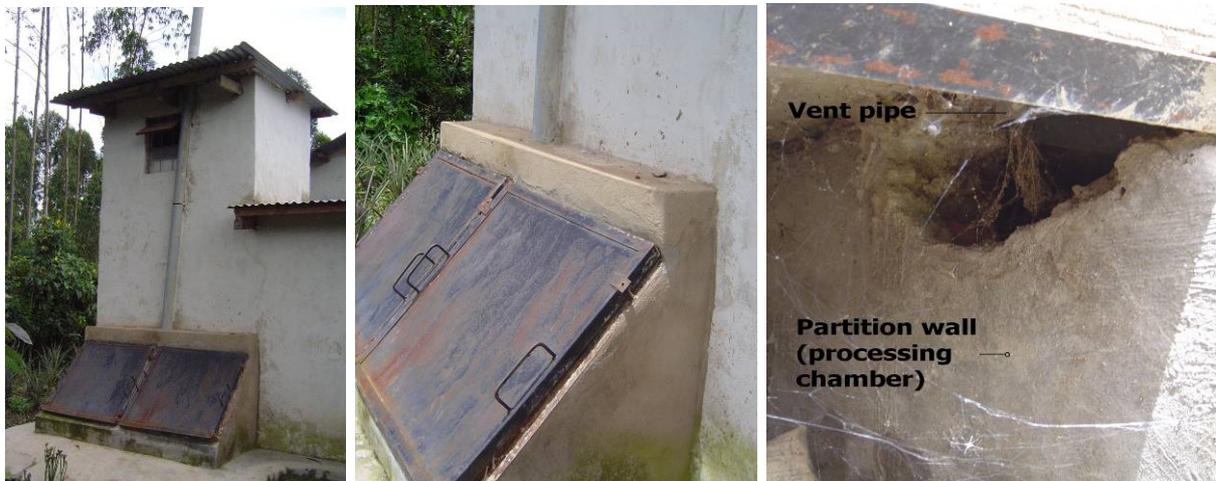
Figure 6.16.: (f.l.t.r.) Rear view (slanting doors; one outside vent pipe). Processing chamber doors. View inside the left Chamber with the bottom of the vent pipe as indicated.
