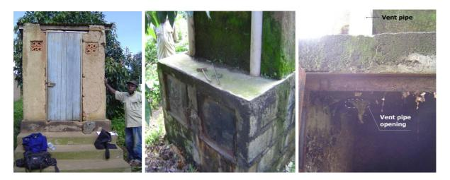
Figure 6.10.: (f.l.t.r.) Front view. Rear view (vertical doors; two outside vent pipes. Detail of the left chamber (vent pipe breakthrough)
