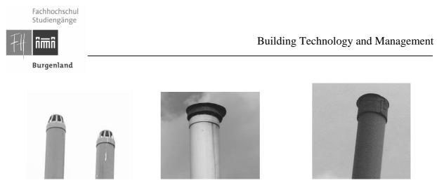
Figure 6.4.: Various rain shelters applied on vent pipes. Left picture represents a cover fitting in Bubaale, Kisoro Rd.; Middle image shows a combination of a cover fitting and a self constructed top piece; Right picture indicates a self construction without any space between the pipe and the shelter.
