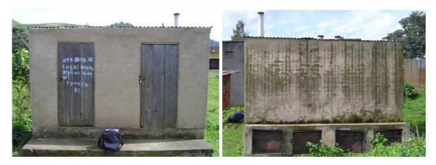
Figure 6.13.: Twin - double vault dry toilet. (f.l.t.r.) Front view. Rear view.
