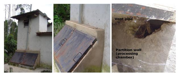
Figure 6.16.: (f.l.t.r.) Rear view (slanting doors; one outside vent pipe). Processing chamber doors. View inside the left Chamber with the bottom of the vent pipe as indicated.
