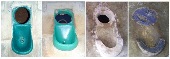
Figure 6.5.: Squatting pans. (f.l.t.r.) 1<sup>st</sup> and 2<sup>nd</sup> picture: Plastic pans in Kalungu. 3<sup>rd</sup> picture: Concrete pan in kisoro. 4<sup>th</sup> picture: Concrete pan with a lid in Kisoro.
