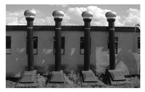
Figure 6.8.: Rear view of an Enviro Loo facility
