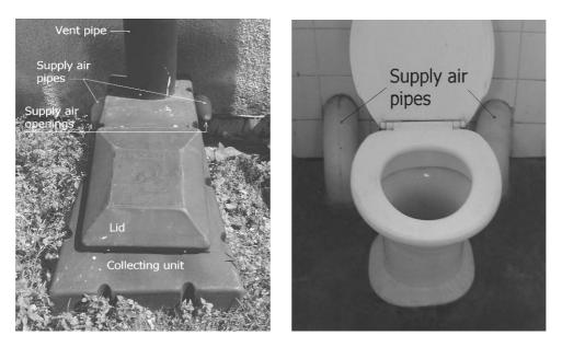
Figure 6.7.: Various parts of an Enviro Loo facility.
