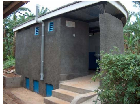
Picture 2: Demonstration urine diverting toilet at “Kalungu Girls Secondary School”, Uganda.
