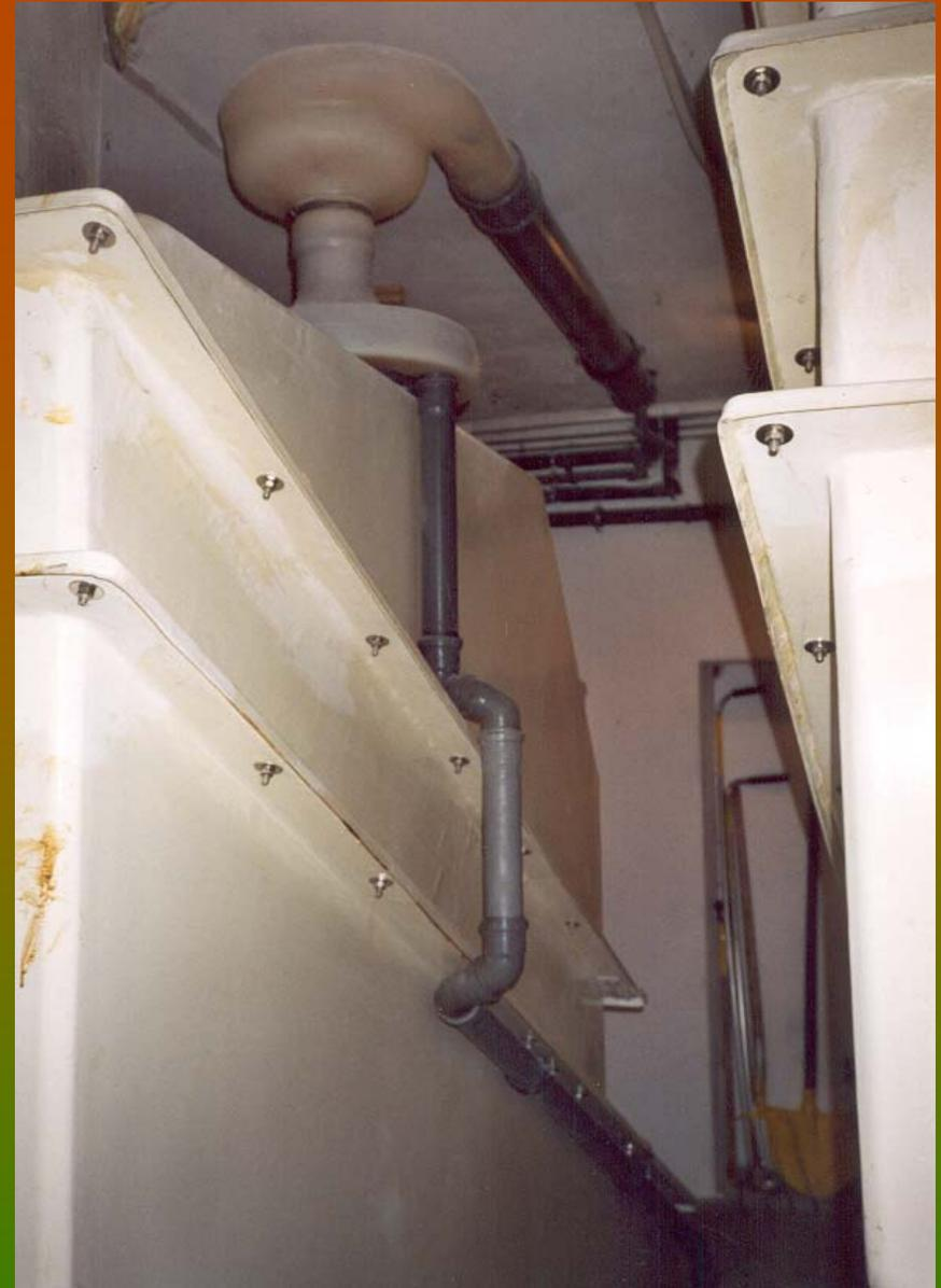
Composting containers and Aquatron separator for flush toilet
