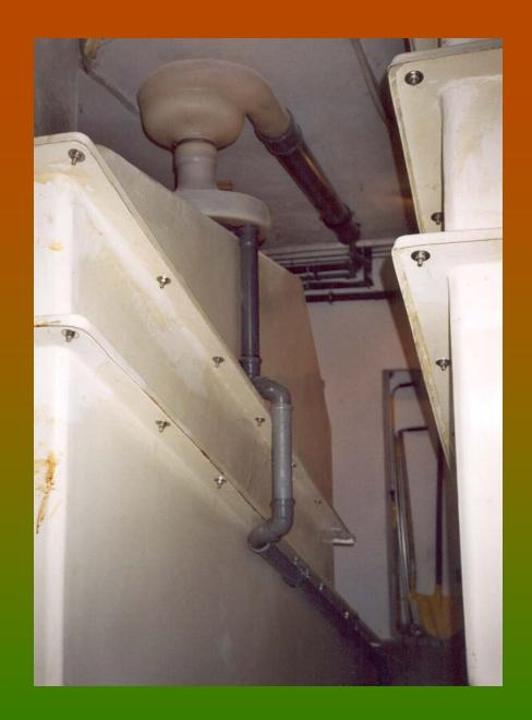
Composting containers and Aquatron separator for flush toilet Berger Biotechnik GmbH, Hamburg
