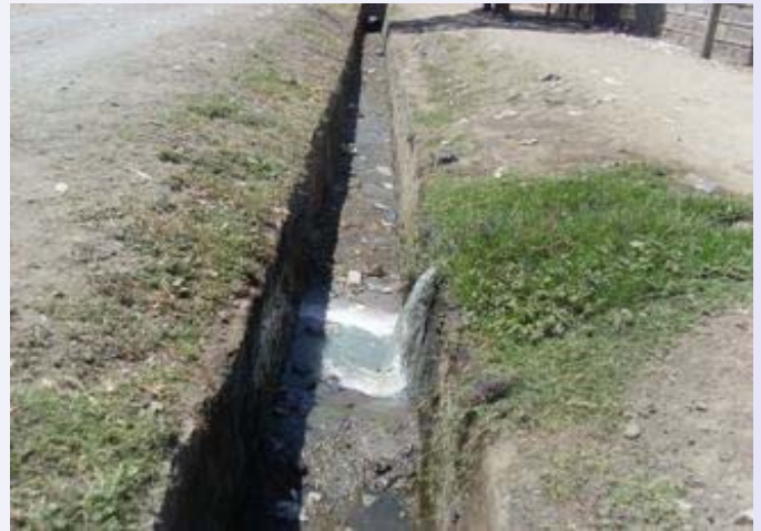
Figure 1: Greywater disposal to storm water drain in Nakuru
