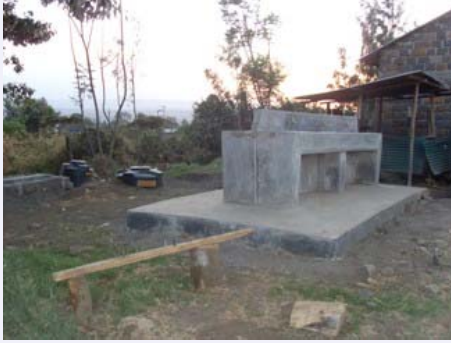
Figure 7: Washing facility- Crater View Secondary School
