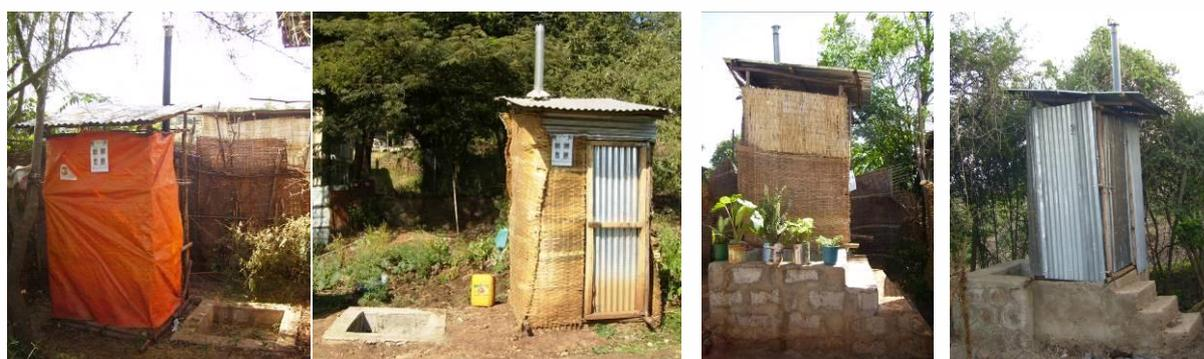
**Figure 3: Fossa alternas constructed for single households.**
