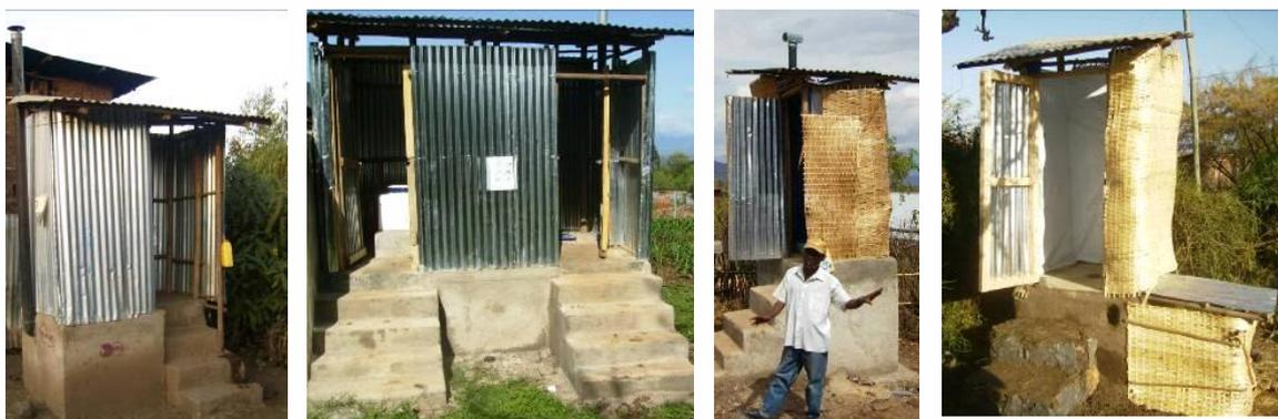
**Figure 2: Some of the UDDTs constructed for single households.**
