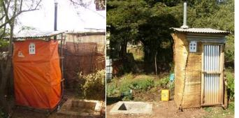
Figure 3: Fossa alternas constructed for single households.
