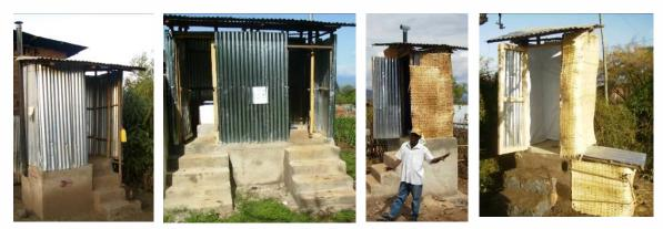
Figure 2: Some of the UDDTs constructed for single households.
