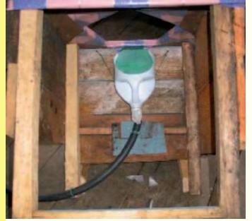
Figure 3: View inside the toilet, showing solidly fixed 1" black hose and easily removable white funnel
