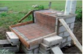
Figure 2: Ferrocement floor and bench before adding concrete. The brown plank forms have no need for holes. (Photo: C. Thibodeau)
