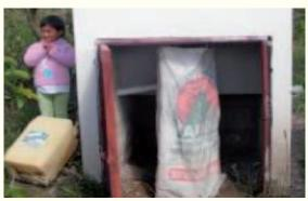
**Figure 4: View of back door.** Note the plastic bottle that collects urine and that the spaces around the door frame should be filled. (Photo: C. Canaday)
