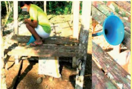
Figure 4: Squatting model UDDT made of palm wood, a funnel and a sack. Privacy walls were added later. Larger funnels may also be preferred
