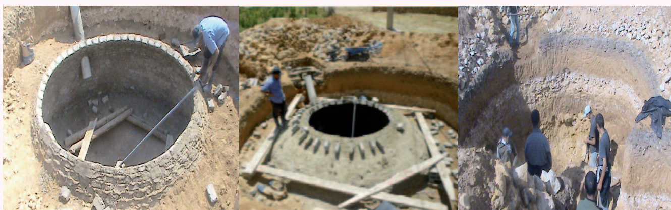
Figure 1 : Biogas plant during construction in Dayet Ifrah village, Morocco (Photos : ABARGHAZ, 2010)
