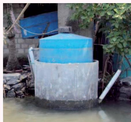
Figure 5: Biogas plant discharging directly into the backwaters
