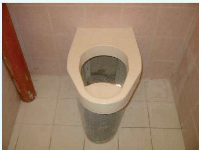
**Figure 3. Toilet seat for a Urine-Diversion Dehydration Toilet (UDDT).**
