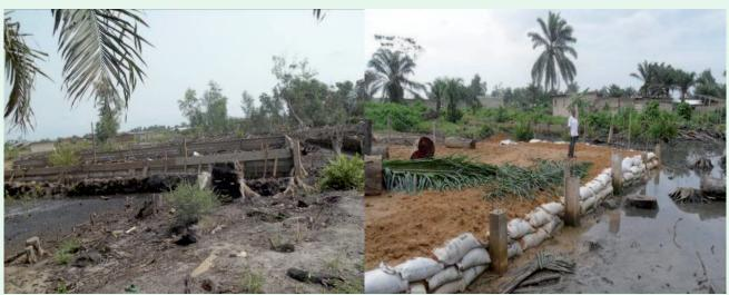
Figure 5: Concrete foundation (on the left) and an earth-filled one in a valley (on the right)
