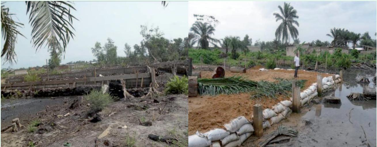
**Figure 5: Concrete foundation (on the left) and an earth-filled one in a valley (on the right)**
