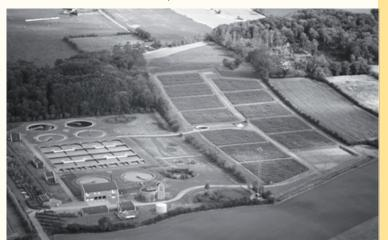
Figure 1: Kolding Sludge Reed Bed System for 125000 PE (September 2000)
