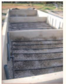
Figure 7. Tertiary VF Sand Filter Cross Photo (2011)
