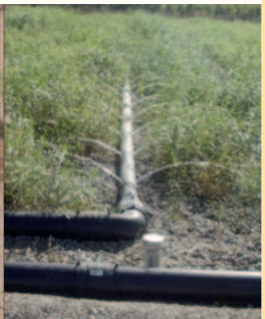
Figure 7: Second stage feeding device (Epur Nature)
