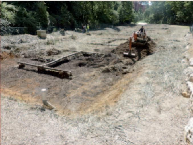
**Figure 12: Sludge removal of the first stage (Roussillon, France) after 14 years of operation**
