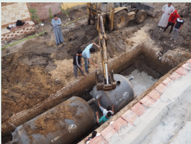
Figure 4. Implementing the EABRA system: Egyptian Anaerobic Baffled Reactor with Aquaponics/Hydroponics. (source: BENAA, 2017)
