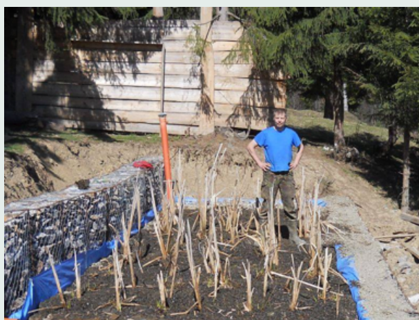
Figure 3 and 4. The first composting toilet and constructed wetland on the Sinevir pass (source: ESF).
