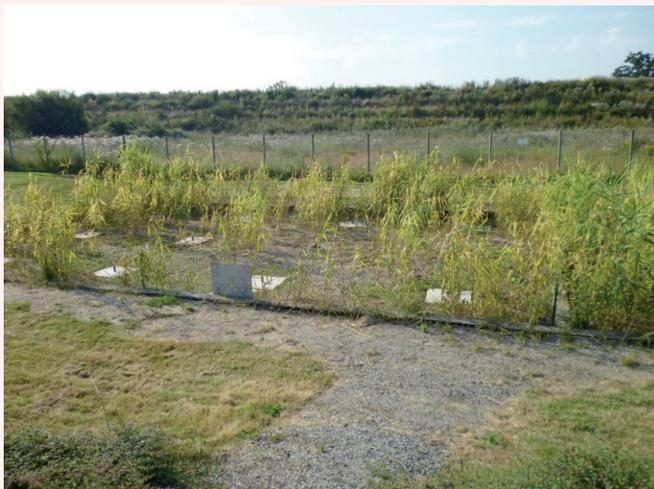
**Figure 4c:** Hauterive second stage French system reed bed, July 2012, showing poor health and disappearance of reeds creating significant reed-free areas (courtesy Joëlle Paing)
