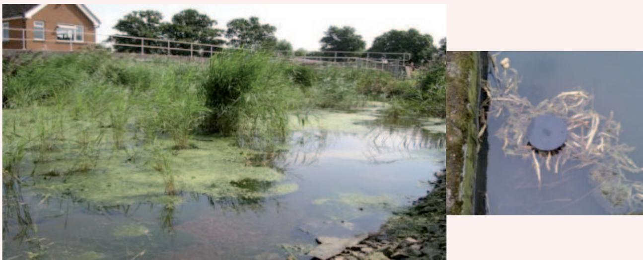
**Figure 1:** Example of subsurface flow wetlands with surface flow during high flow conditions. The water flows preferentially over the top of the bed and will result in partially treated water exiting through the overflow pipe and blending with the treated effluent at the final collection point.
