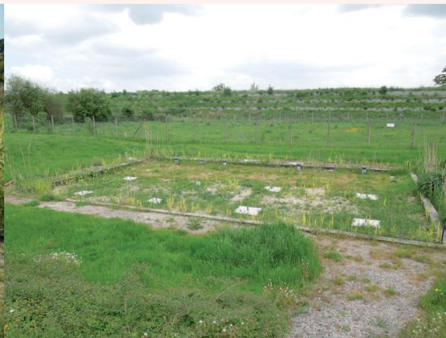
**Figure 4d:** Hauterive second stage French system reed bed, May 2013, almost complete disappearance of reeds within three years of first yellowing, with replacement by “weeds” (courtesy Joëlle Paing)
