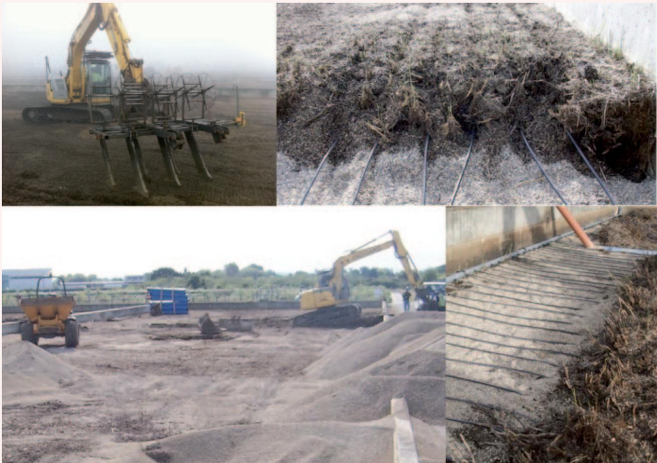
**Figure 3: Retrofit of an aeration system into an existing treatment wetland at Mayfield Farm, UK.**
