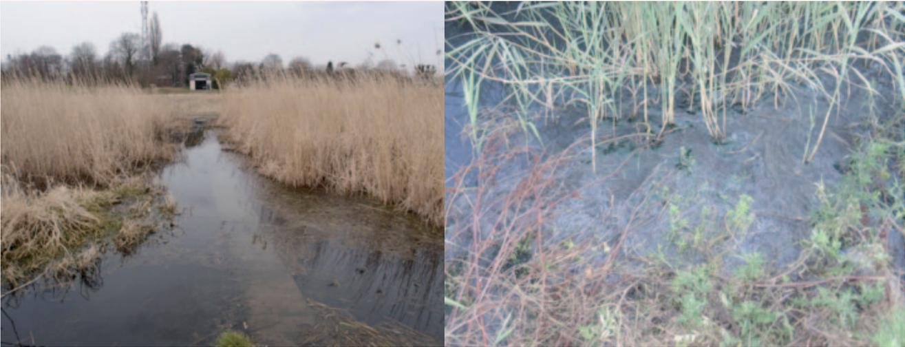
**Figure 4: Examples of clogged horizontal flow wetlands (a) Hydraulically linked UK tertiary wetland cells and (b) Surface ponding and hydrogen sulfide generation in secondary wetland in Italy. Picture (b) courtesy of IRIDRA Srl.**
