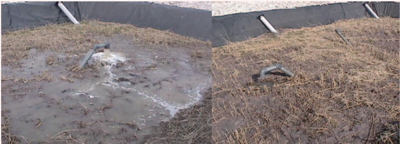
**Figure 2:** Example of 1st stage VF Wetland with ponding during feeding. The water flow preferentially over the top of the bed around inlet points and the percolates.
