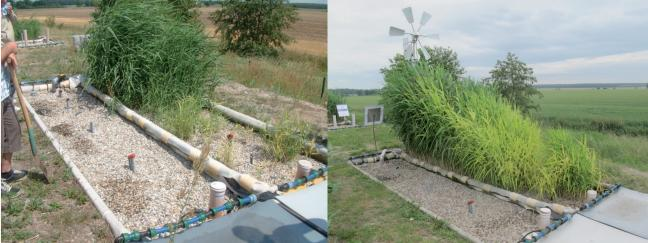
Figure 5a: Langenreichenbach horizontal flow forced aeration reed bed, receiving settled effluent: tall, green, dense reeds near inlet; short, yellow reeds further from inlet (1Jul11)
