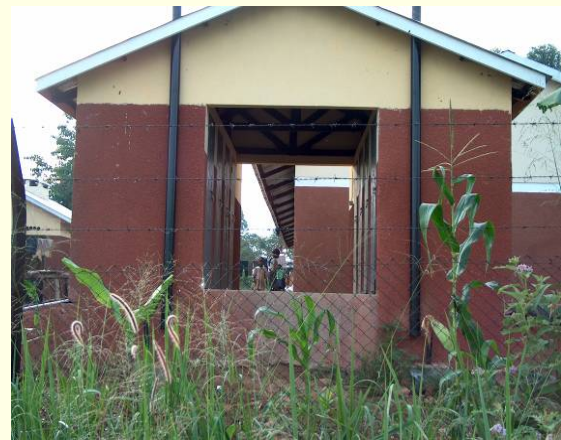
Figure 1: Urine diverting dry toilets in Maracha Hospital.
