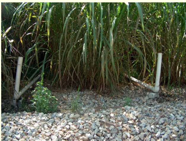
Figure 7: Vertical-flow constructed wetland.
