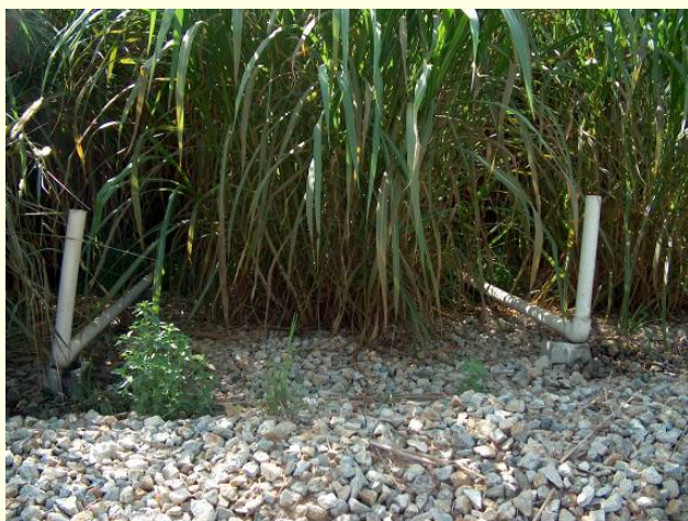
Figure 7: Vertical-flow constructed wetland.
