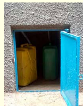
Figure 3: Wooden collection container for faeces and urine collection in 20l jerry cans.
