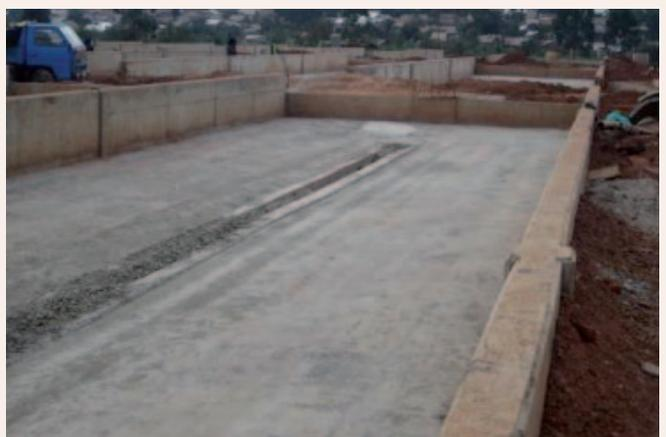
**Figure 3: Drying beds in construction at the new faecal sludge treatment plant in Kampala.**
