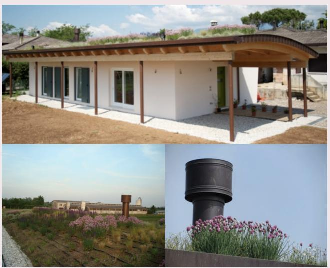
Figure 5: Green roof at the wooden house in Treviso, Italy
