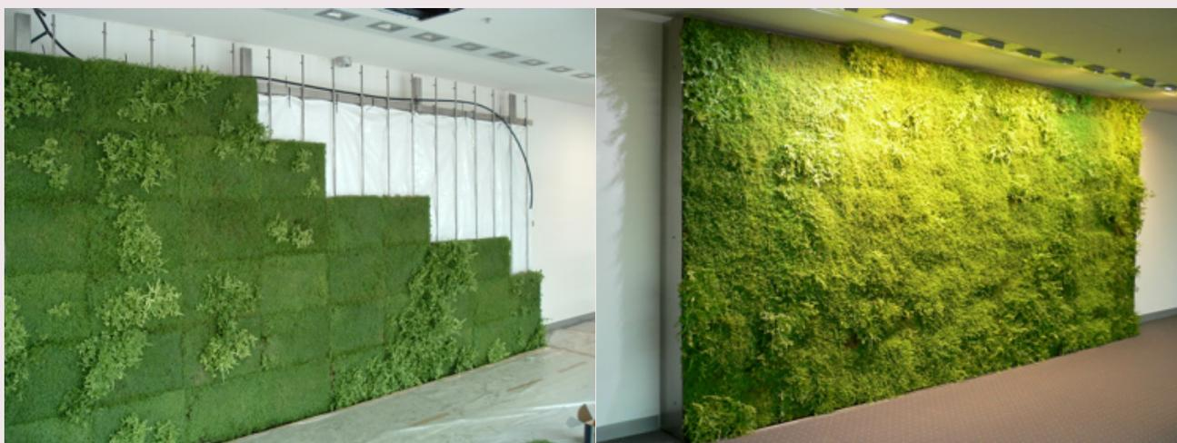
**Figure 2.** Green Wall Sparkassa Ingolstadt: modular system (left) and later the connate plates (right) (photo by B. Häring)
