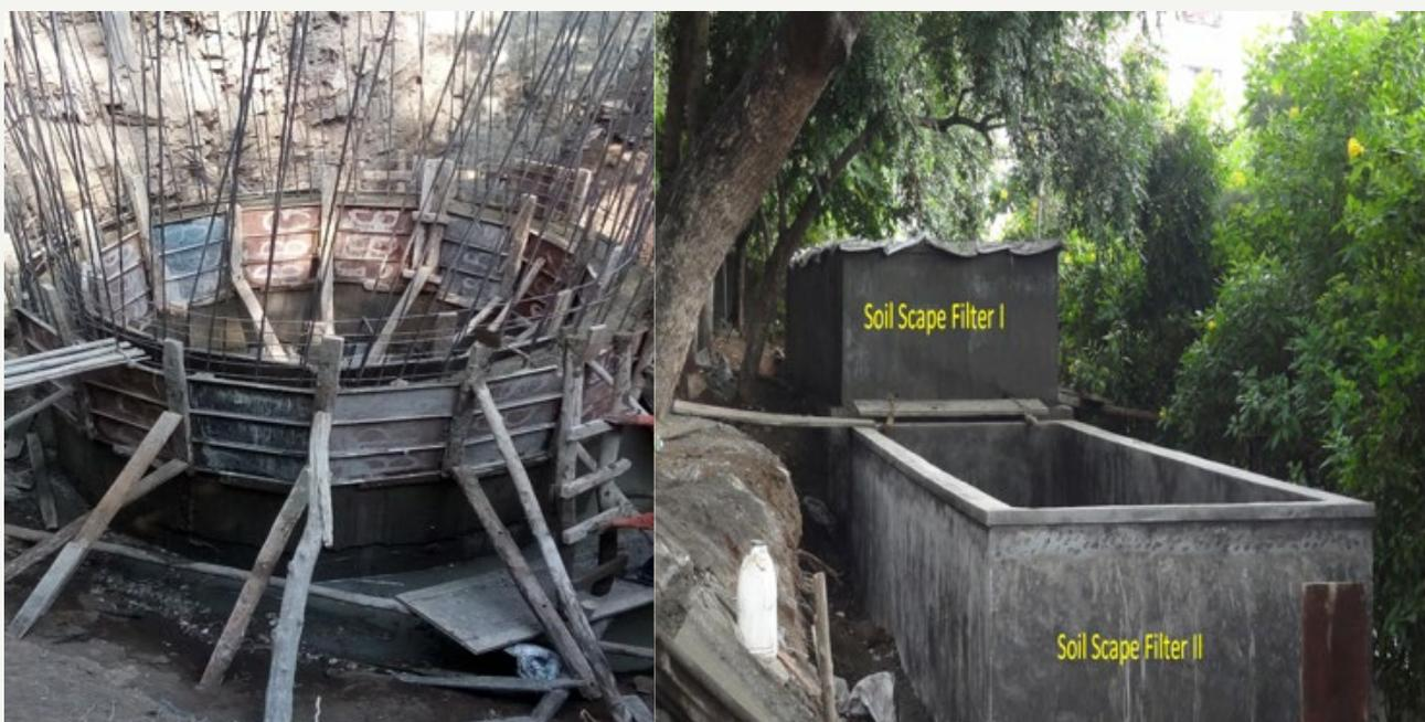
Figure 6 - Construction of intake well (left) and soil scape filter beds (right).
