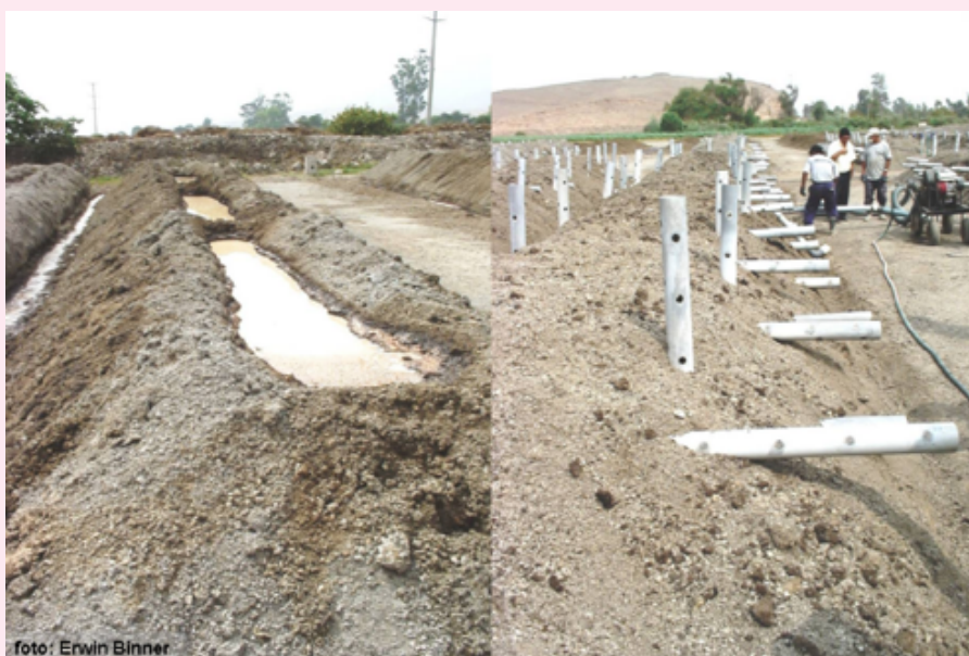
Figure 5. Composting of paper-mill sludge – example for too less free air space.
