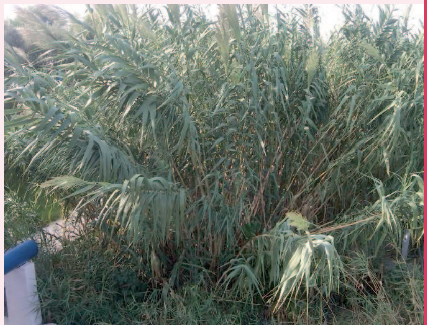
Figure 2: Decentralized system for rural community: Constructed wetland system in Tunisia.
