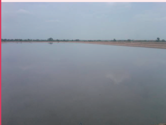
Figure 3: Large space requirement for pond systems: Ouagadougou WWTP (Burkina Faso); Treating 96 m 3 /h of domestic and industrial wastewater.
