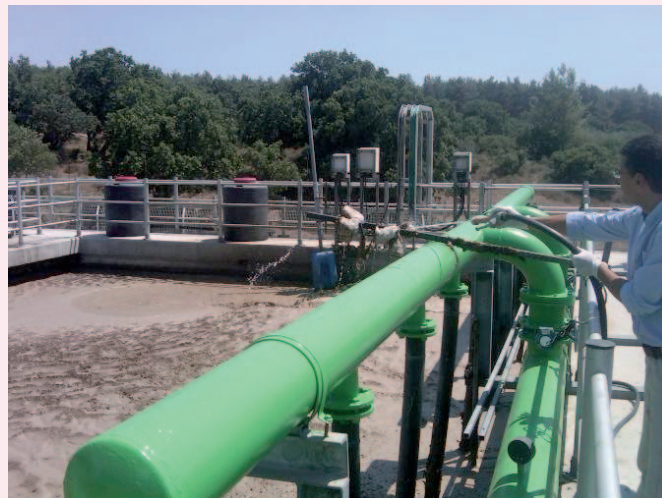
Figure 4: Domestic MBR plant with impact from olive oil production wastewater (inhibition due to phenolic compounds; Israel).
