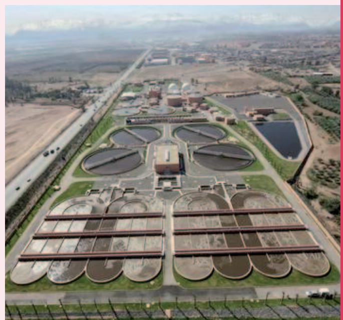
Picture 4: Marrakech Aerobic WWTP with sludge digestion and methane production for energy cogeneration
