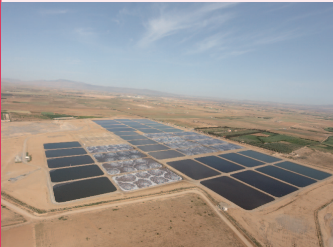
Picture 2: Largest aerated lagoons in Morocco (Oujda city)
