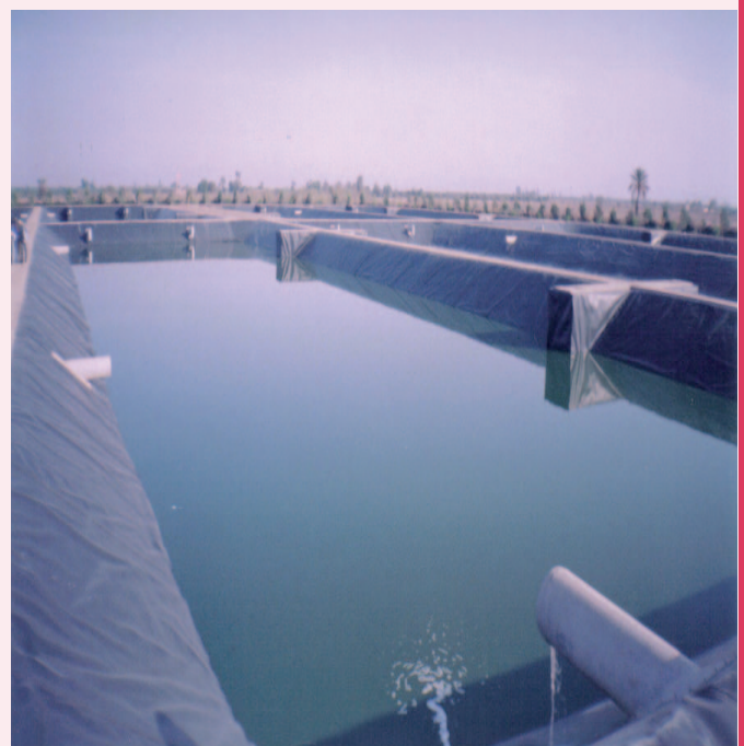
Picture 1: Natural lagoons for wastewater treatment plant of the Saada commune (Peri-urban area of Marrakech city)
